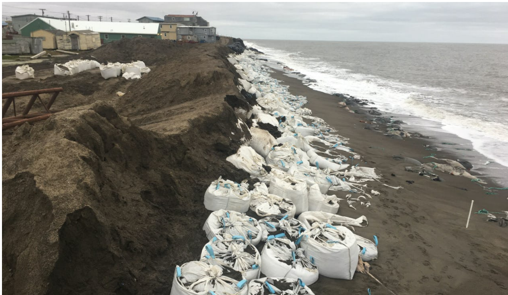
Temporary coastal erosion control using supersacks in Utqiagvik, Alaska, August 28, 2019. Photo: Louise Farquharson
