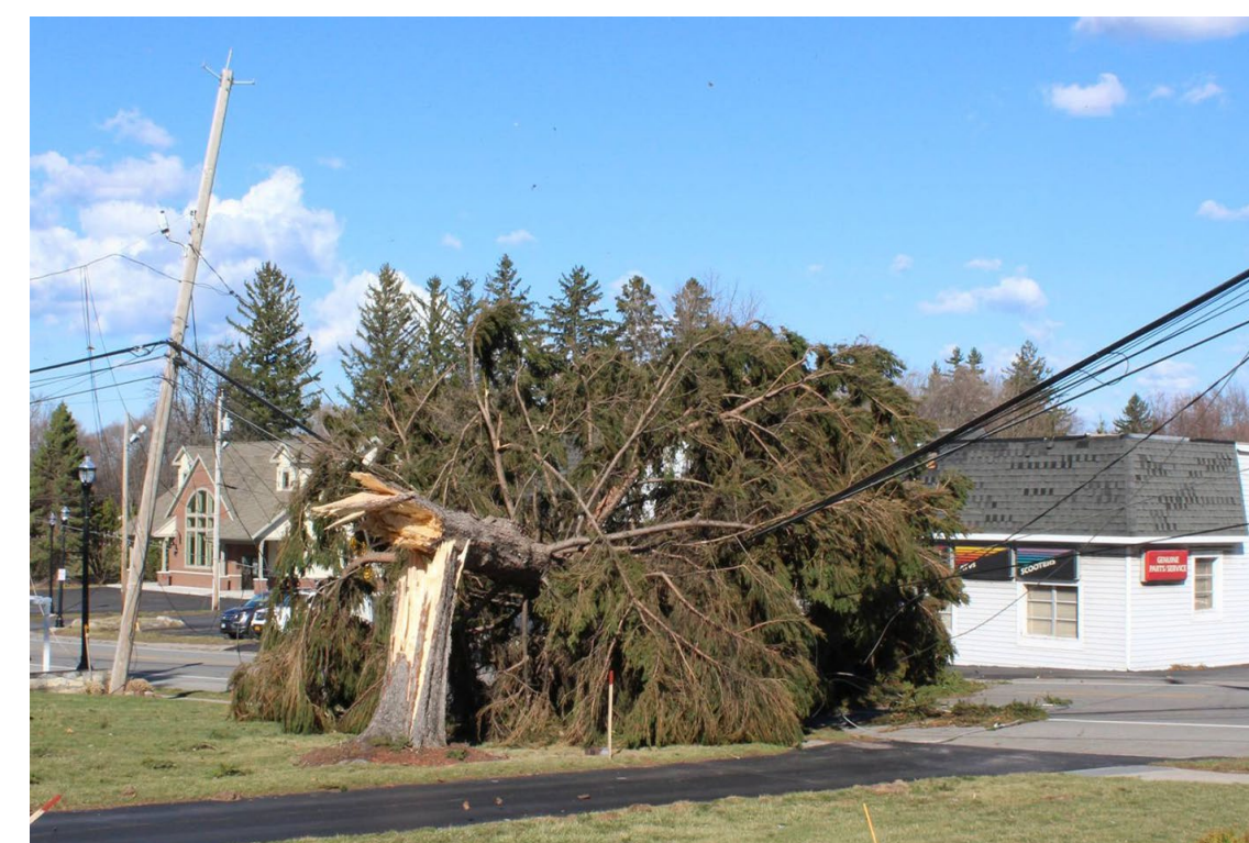
Figure 3. Falling trees and power lines.
